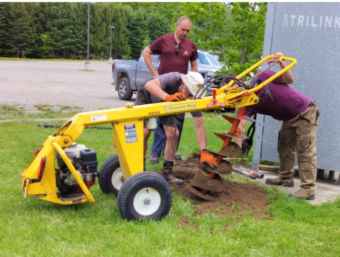
(Below) Another picture of the engineer and contractor digging a test hole at the tower site, courtesy of Neil VA3NH .
